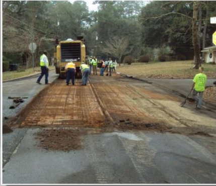
Milling and Resurfacing
