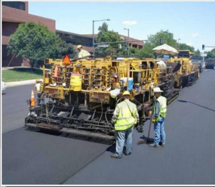
Hot in Place Recycling
